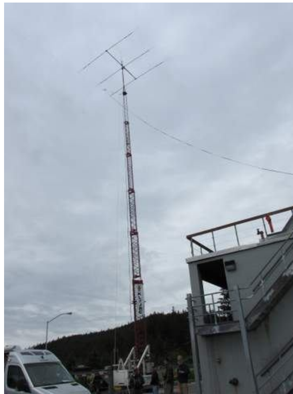
KL7JRC Motorized 100 foot tower
