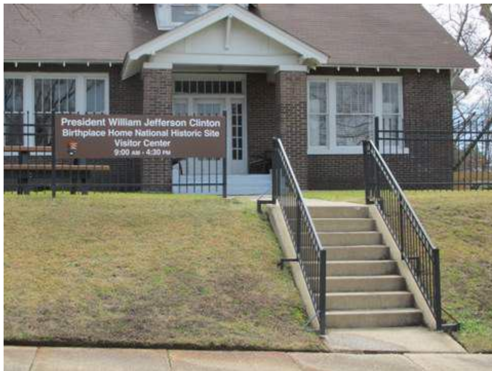
Visitor Center Note picnic table on left
